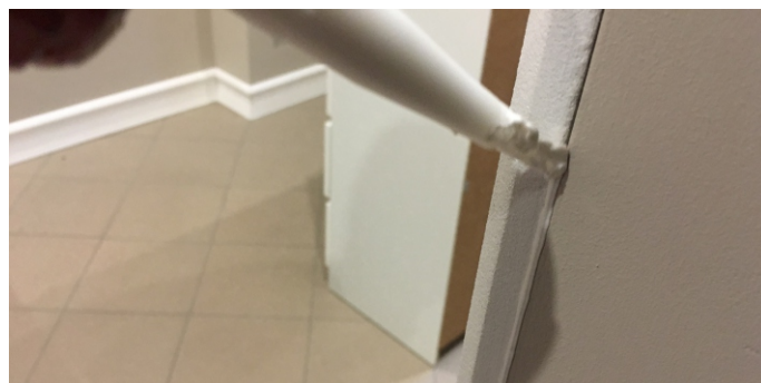
Photo 9. Sealing the Connection of Wall and Moulding
