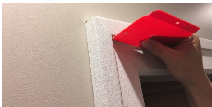
Photo 8. Joints Grouting
