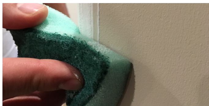
Photo 10. Cleaning the Joints
